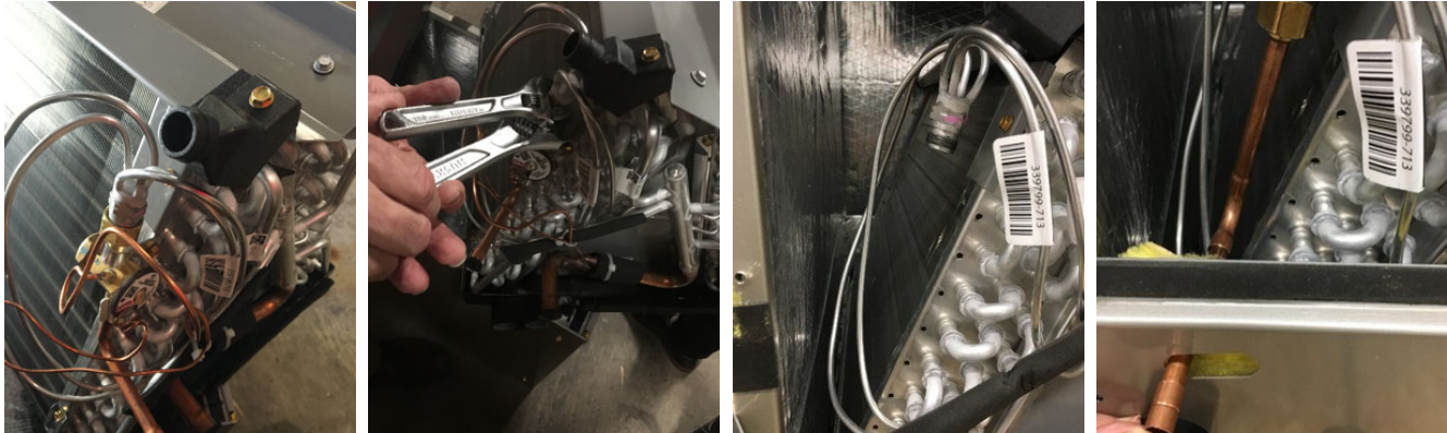
Fig. 14 — Piping Adapter Replacement
