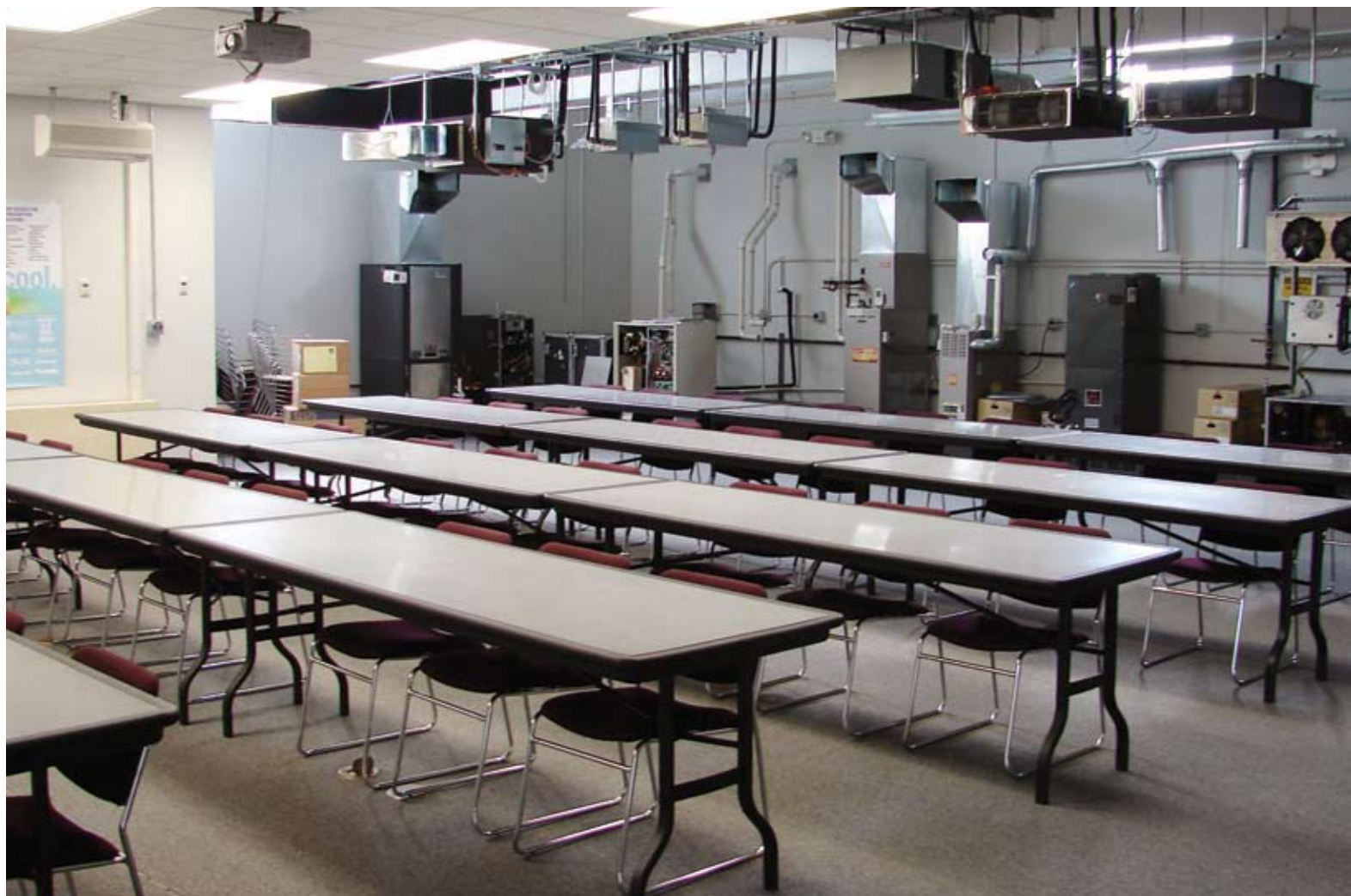
The large training facility at Behler-Young's New Hudson, Mich., location allows HVAC contractors to send employees to regularly scheduled classes in the same building they pick up their parts and equipment.
